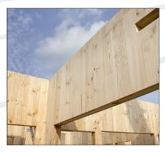
Various products where timber lamellas are connected and glued on top of each other. Lamellas are stacked on top of layer below and lamellas are stacked 90 degrees on a prior level. The glue is applied on the horizontal layer.
